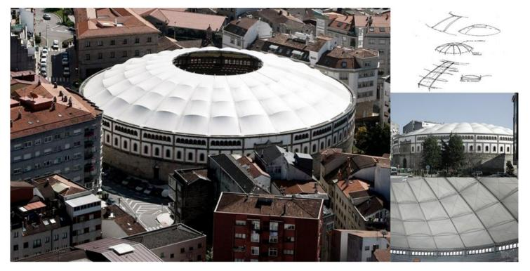
The roof structure of the bullring in Pontevedra is conceived as a shell in form of a semi-spheroidal segment 69.0m in diameter with a ring-shaped central opening 25.0m in span.
